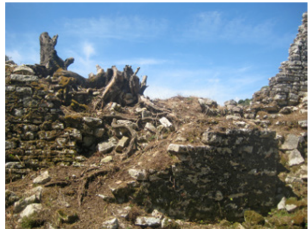
Fig. 3. The roots and a massive trunk inserted in the structure of a medieval wall
