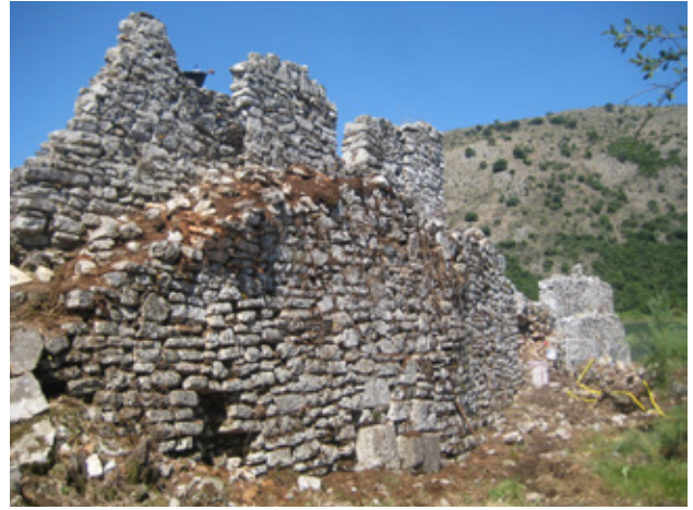
Fig. 9. Documentation of the construction technique on the northwest spur and the presence of mud in the inner part of the structure
