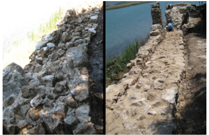
Fig. 7. Fragment from the Circuit wall line; after its cleaning from the organic remains and vegetation and after its restoration and consolidation
