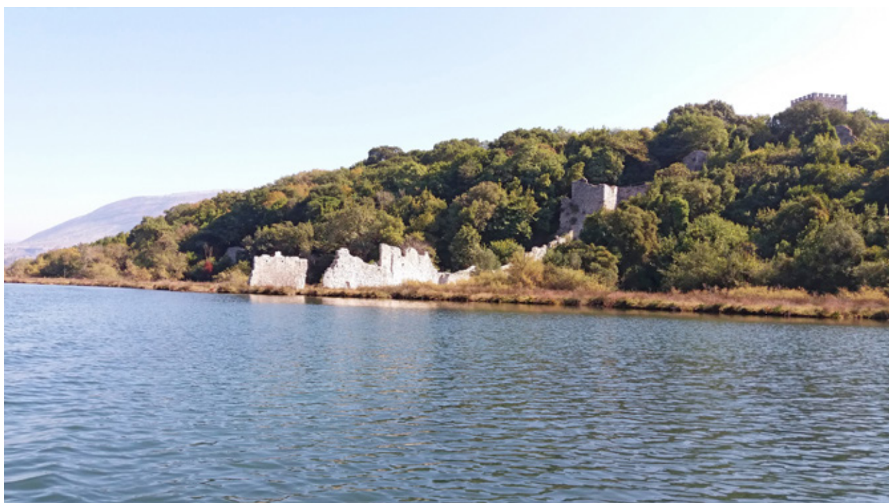
Fragment of the circuit wall (Northwest Spur) along Butrint's Lake after restoration
