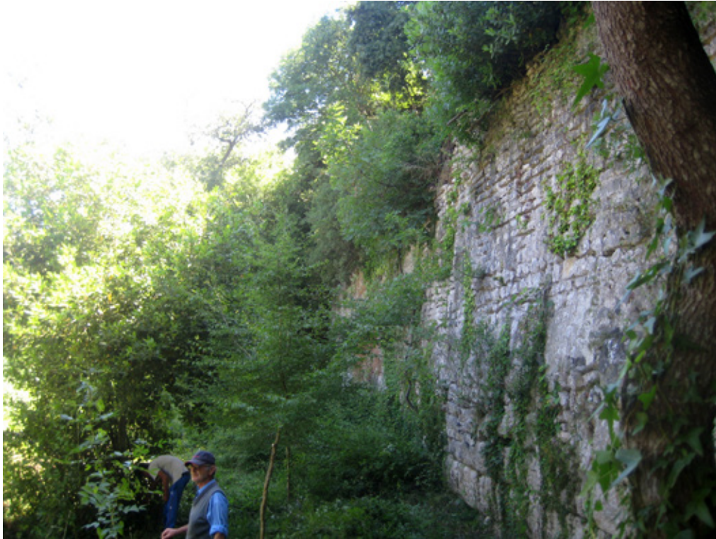
Fig. 2. Presence of vegetation near and on the wall's structures
