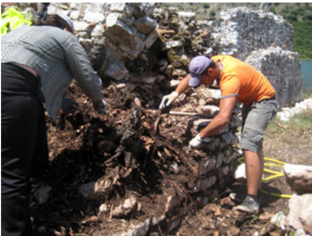
Fig. 5. Mechanical cleaning of deteriorated roots of the trees and other organic remains
